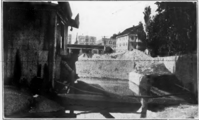
Concrete Settling Pond
